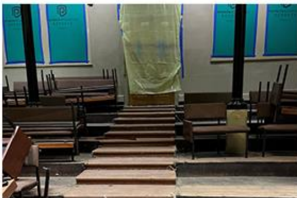
Flooring stripped out to upper section of the lower auditorium.
